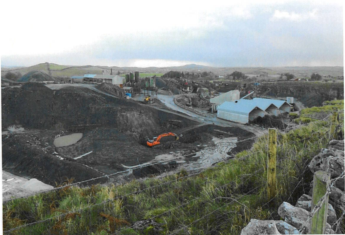
November 2015 – quarrying in south quarry
