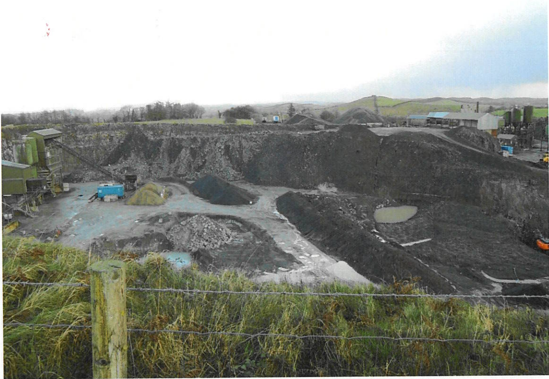
November 2015 – quarrying in south quarry
