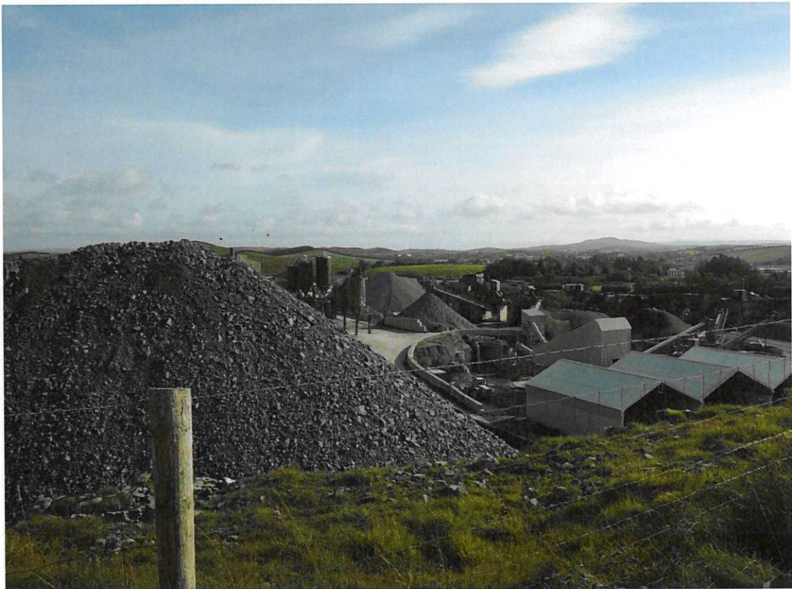
October 2013 - materials excavated in the north quarry stockpiled in the south quarry
